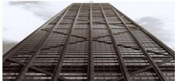
Fig 4: Cross bracing in building
